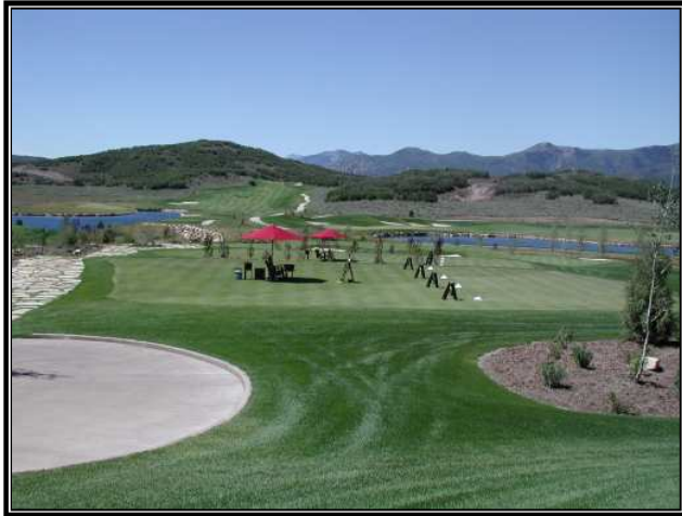
Finished practice tee box.
