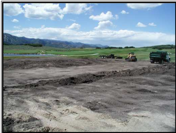
Renovating existing green and tee box.
